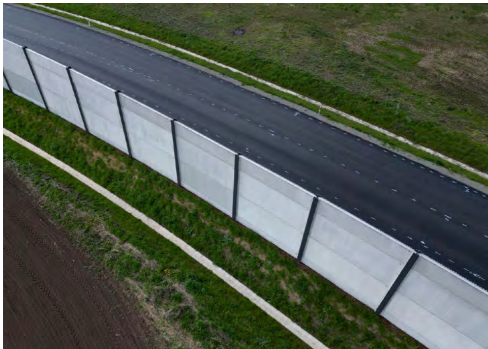
Figure 17. Noise Barrier Wall
