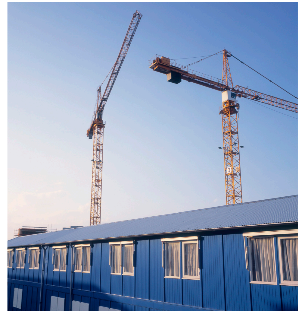
Figure 58. Examples of Temporary Construction Compounds
